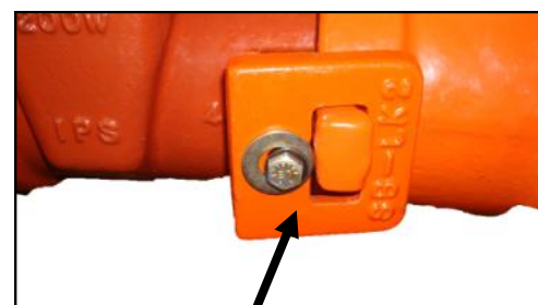
Picture of properly installed SB-LK link
